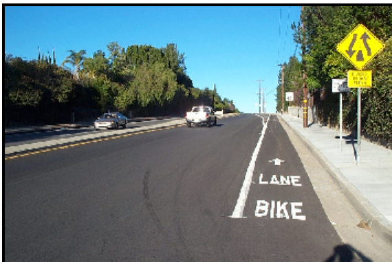
Existing Middle Segment of Zone 1
