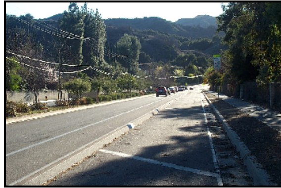
New Asphalt Berm near Daguerre Drive
