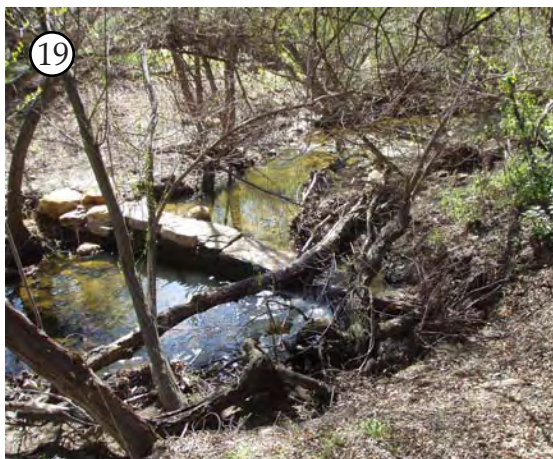
Photo: J.Hall Irrigation dam from the early 1900s. The dam is used as a footbridge connecting a trail from the Masson House to MRT offices.
