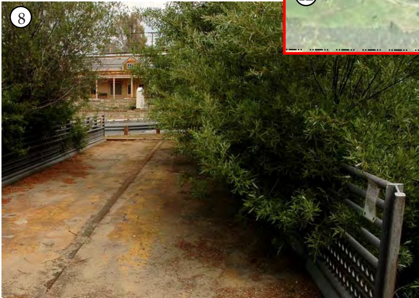
Access to the trails of Headwaters Corner from Old Topanga Canyon Road uses this bridge, built in 1995 from recycled materials: flatbed railcars, oil casing pipe, WWII landing mat and used railroad track. View is towards Old Topanga Canyon Road.
