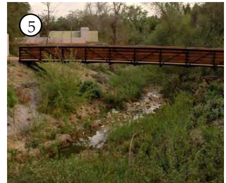
5 Dry Canyon Creek restoration area with MRT office in background. Restoration removed concrete and asphalt and implemented soil bioengineering of streambanks with willow cuttings.
