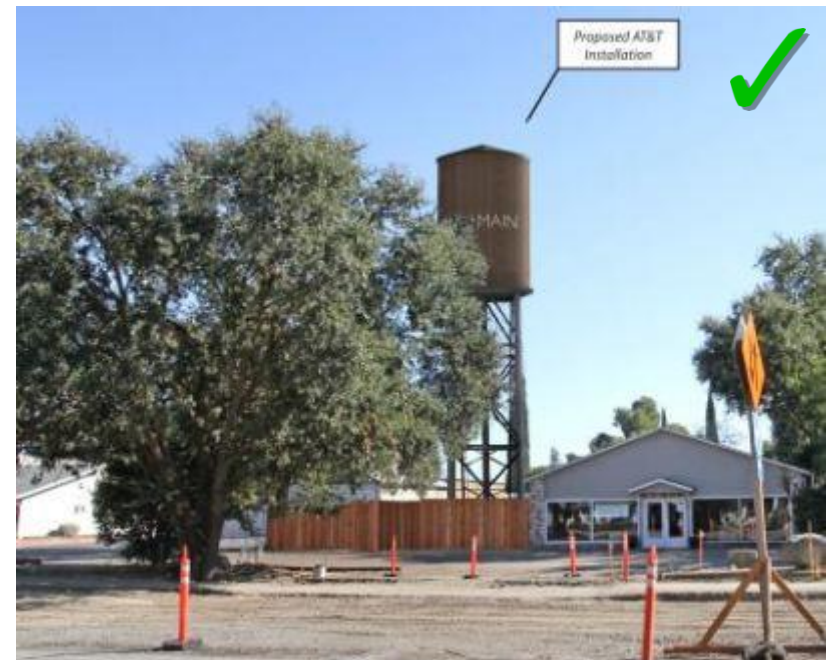
Figure 19: Successful rendering from project outside Calabasas; all equipment screened within faux water tank.
