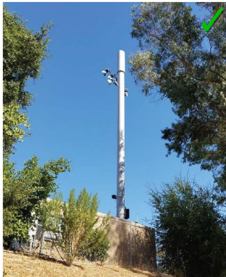
Figure 21: Successful example from facility at Calabasas High School; all equipment screened, and radome camouflaged to match pole.
