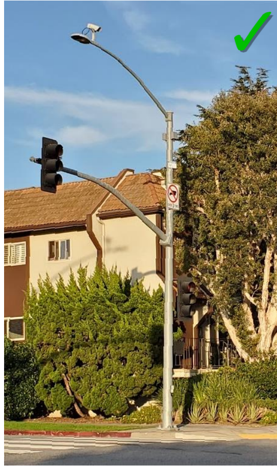
Figure 26 Successful example outside Calabasas; minimal pole mounted equipment, no ground mounted equipment.
