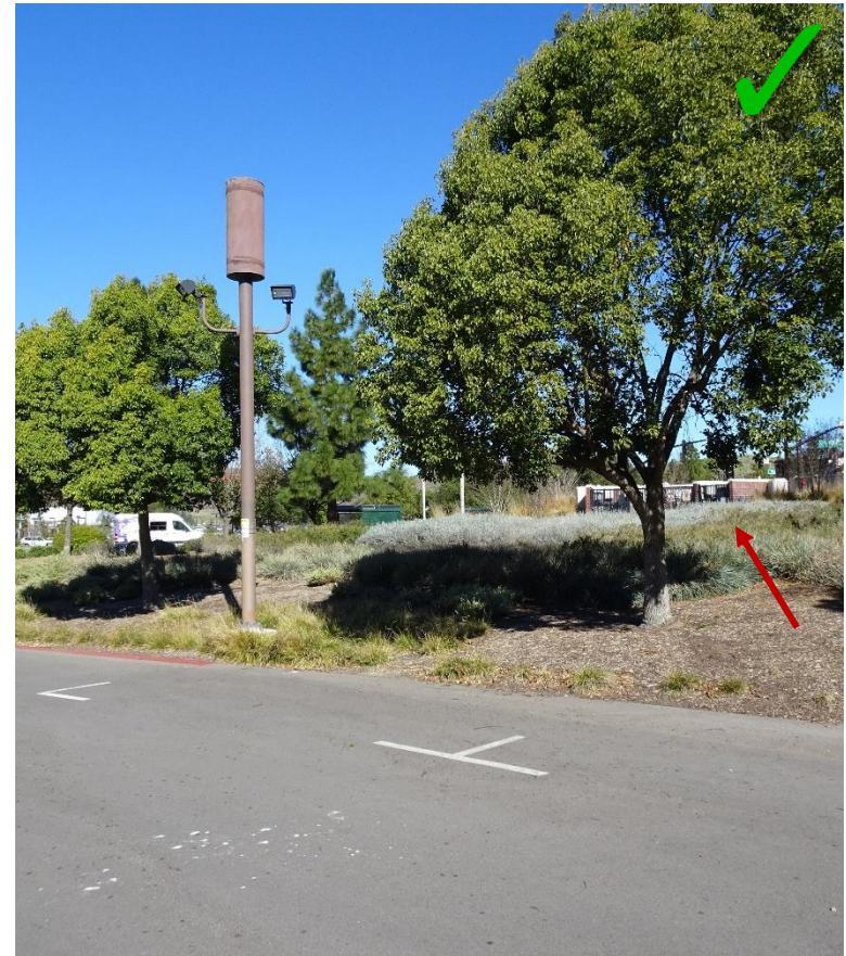
Figure 17: Successful example outside Calabasas; all antennas contained within radome and ground mounted equipment is screened (see red arrow), compatible in scale with surroundings.
