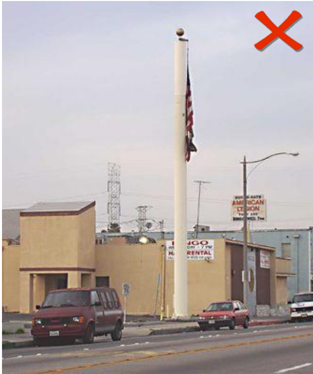
Figure 14: Unsuccessful example outside Calabasas; although facility is camouflaged, pole is not compatible in size (both height and diameter) or scale with surroundings.
