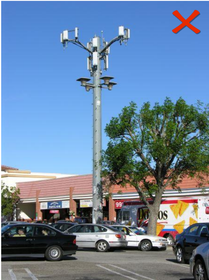
Figure 16: Unsuccessful example outside Calabasas; facility not camouflaged, pole not compatible in size or scale with surroundings.
