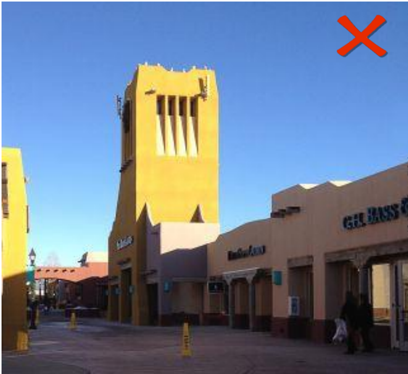
Figure 8: Unsuccessful example outside Calabasas; antennas mounted on the facade of the tower feature rather than inside the feature, and the tower feature itself is not compatible in scale or design with surrounding context.
