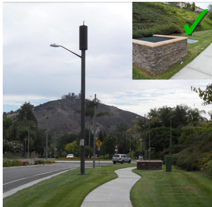
Figure 23: Successful example in Calabasas; equipment concealed within radome ground mounted equipment screened behind rock wall enclosure.
