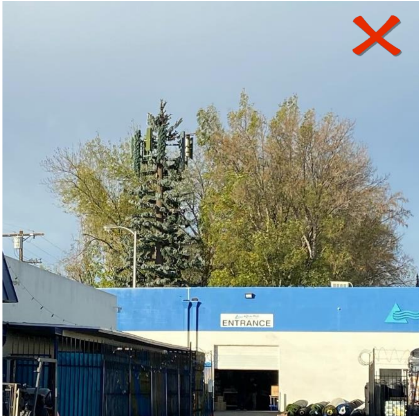
Figure 12: Unsuccessful example outside Calabasas; faux tree species is not compatible with surrounding trees, and equipment is not properly camouflaged—antennas still visible.
