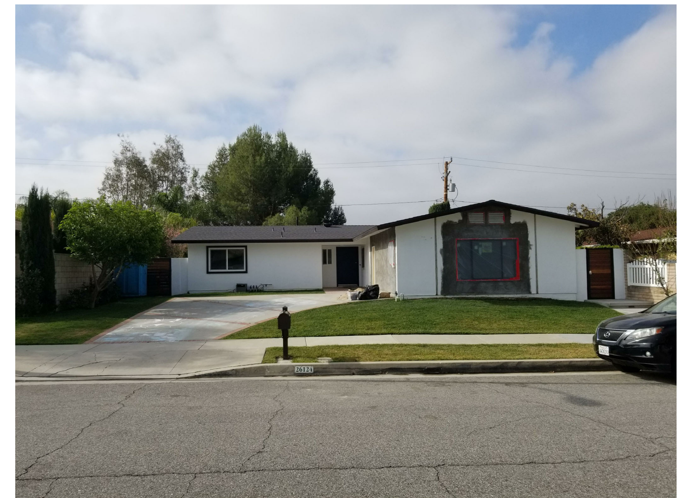
EXISTING STREET VIEW (JADU UNDER CONSTRUCTION)
