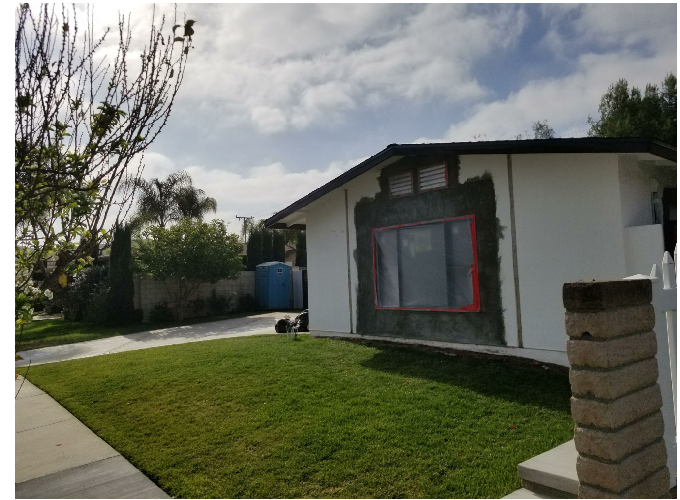
EXISTING STREET VIEW (JADU UNDER CONSTRUCTION)
