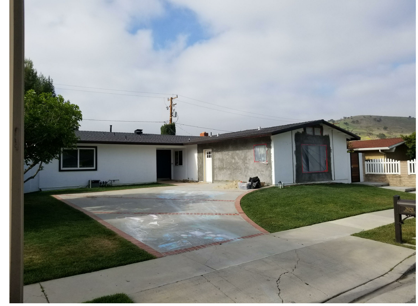
EXISTING STREET VIEW (JADU UNDER CONSTRUCTION)
