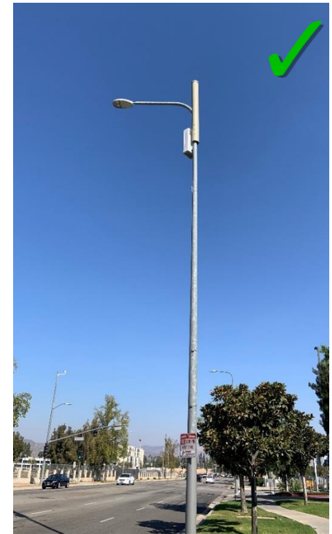
Figure 24: Successful example outside Calabasas; equipment and antennas concealed.
