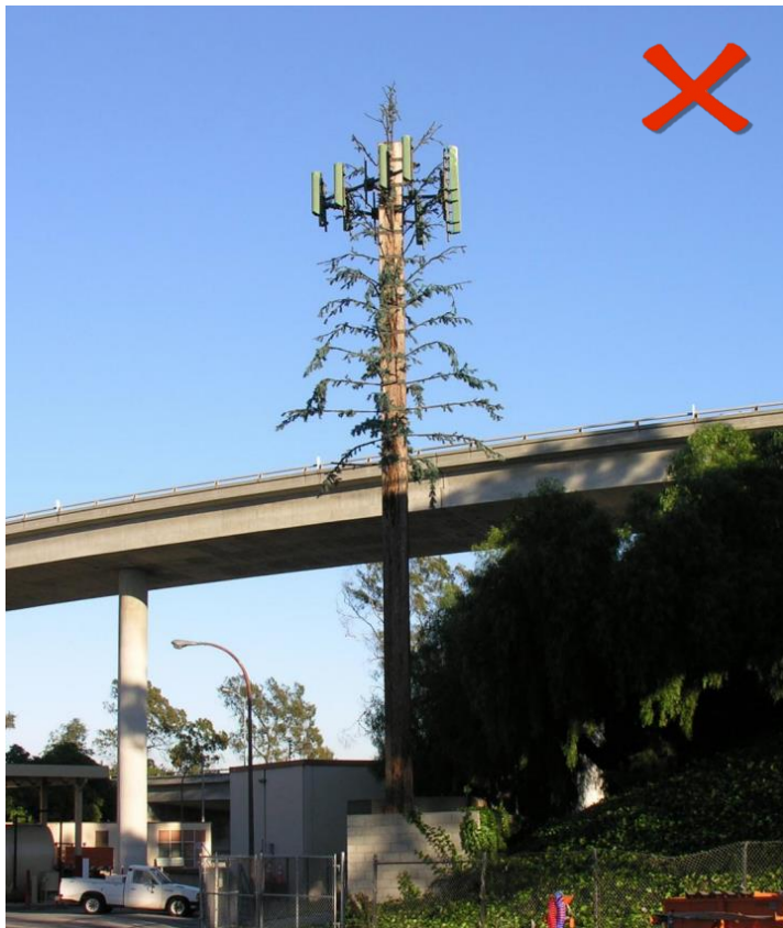
Figure 10: Unsuccessful example outside Calabasas; does not blend in with surroundings and poor tree design.
