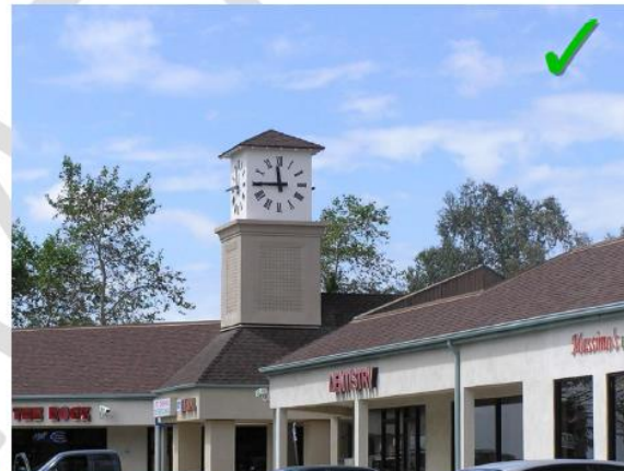
Figure 9: Successful example outside Calabasas; all equipment concealed within feature and is architecturally compatible with existing roof.
