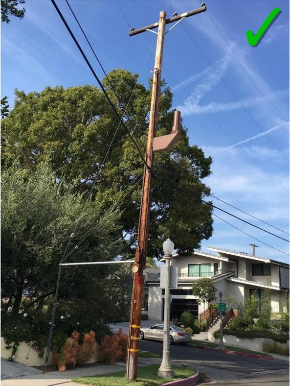
Figure 32: Successful example outside Calabasas; equipment is minimal, and painted to match pole.
