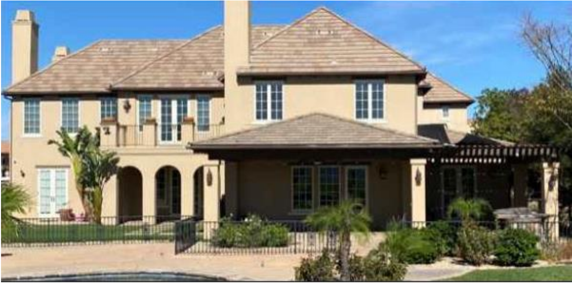
Rear of existing house
