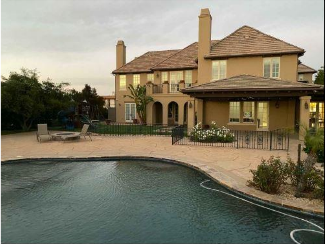
Rear of existing house 2
