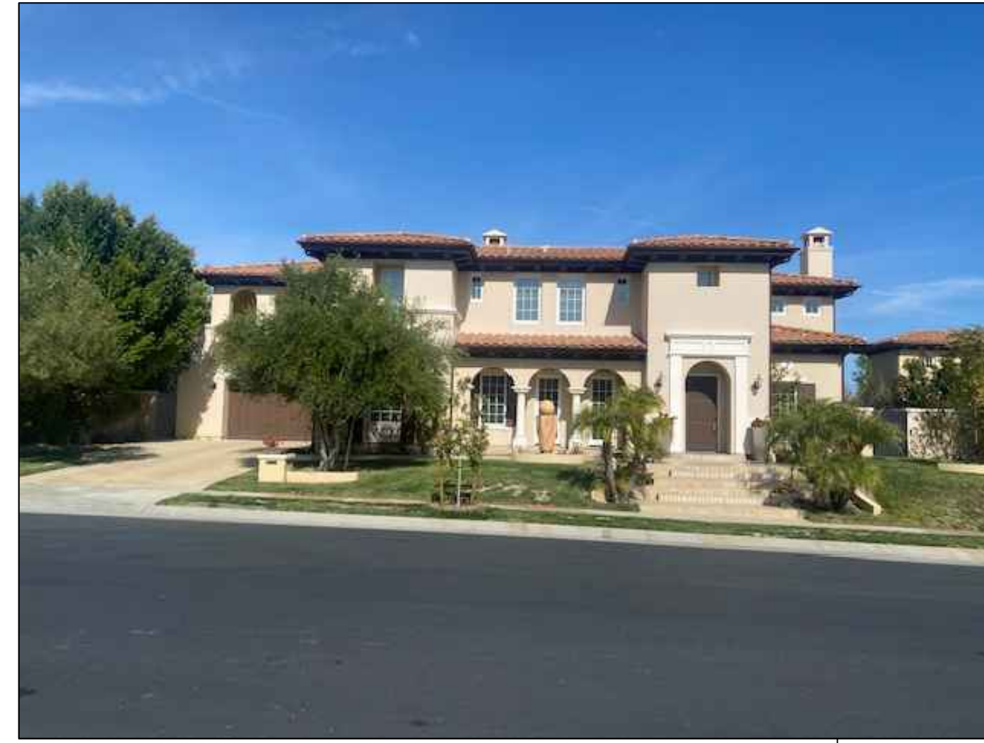
25471 PRADO DE AZUL (ACROSS THE STREET - 4 DOORS AWAY) Building Area: 6,745 SF. Lot Area: 14,299 SF. FAR: 0.47
