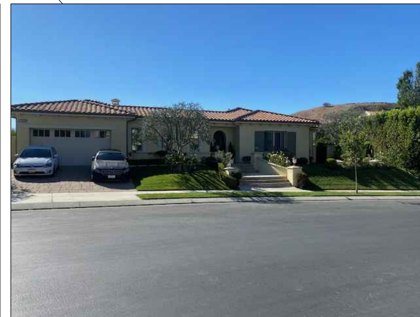
25520 PRADO DE AZUL (HOUSE TO THE RIGHT) Building Area: 5,802 SF. Lot Area: 20,956 SF. FAR: 0.27
