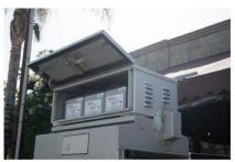
The internal mounted battery solutions place them on a tray within the cabinet so there will be nothing visible externally to how the cabinets currently look.
