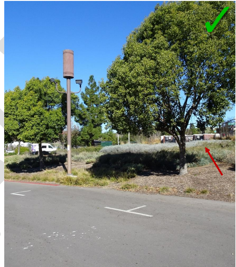
Figure 17: Successful example outside Calabasas; all antennas contained within radome and ground mounted equipment is screened (see red arrow), compatible in scale with surroundings.
