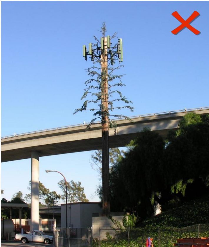
Figure 10: Unsuccessful example outside Calabasas; does not blend in with surroundings and poor tree design.
