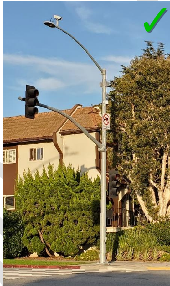
Figure 26 Successful example outside Calabasas; minimal pole mounted equipment, no ground mounted equipment.
