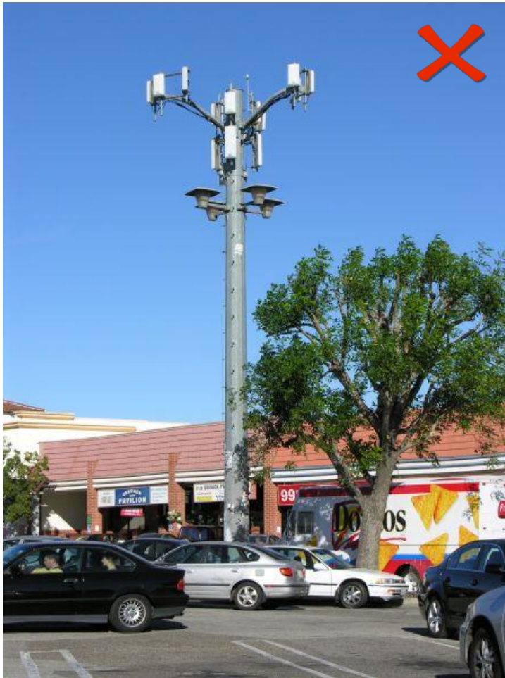
Figure 16: Unsuccessful example outside Calabasas; facility not camouflaged, pole not compatible in size or scale with surroundings.
