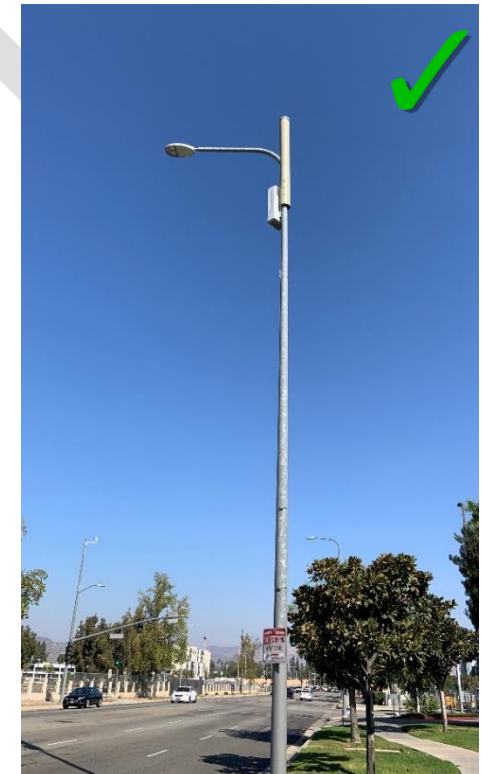
Figure 24: Successful example outside Calabasas; equipment and antennas concealed.
