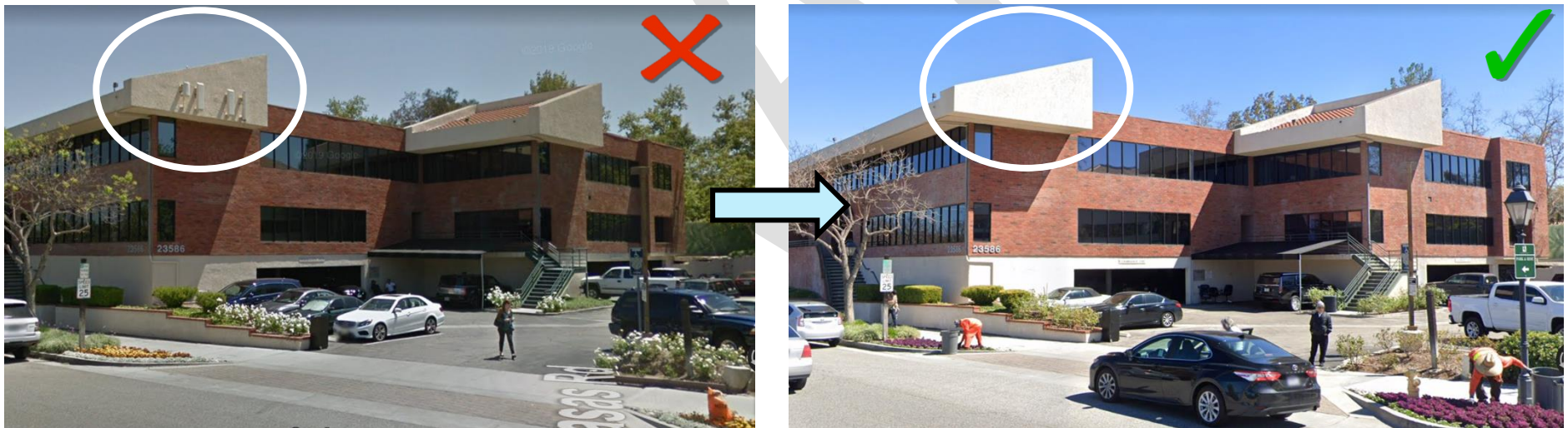
Figures 2 & 3: Before-and-after images showing successful faux façade element constructed out of fiberglass to screen existing antennas.
