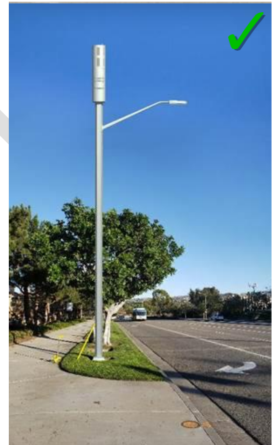
Figure 27: Successful example outside Calabasas; equipment and antennas concealed, no ground mounted equipment.
