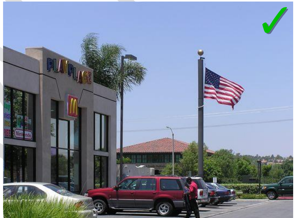
Figure 15: Successful example outside Calabasas; pole is compatible with surroundings in scale and design, and facility is properly camouflaged.
