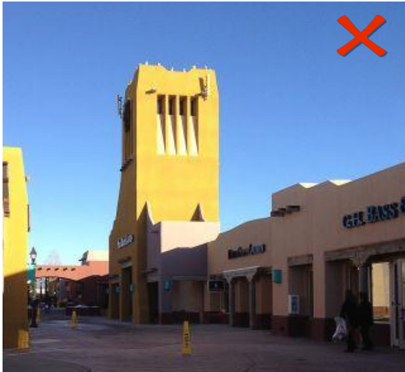
Figure 8: Unsuccessful example outside Calabasas; antennas mounted on the facade of the tower feature rather than inside the feature, and the tower feature itself is not compatible in scale or design with surrounding context.
