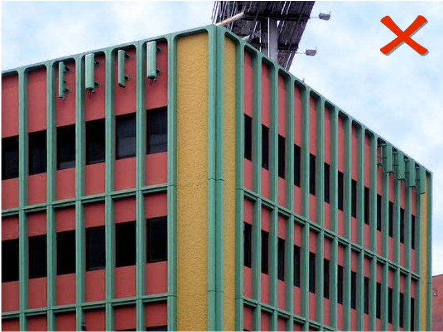
Figure 6: Unsuccessful example outside Calabasas; antennas are painted to match building elements but are not fully screened/camouflaged. Would not be considered a stealth facility.
