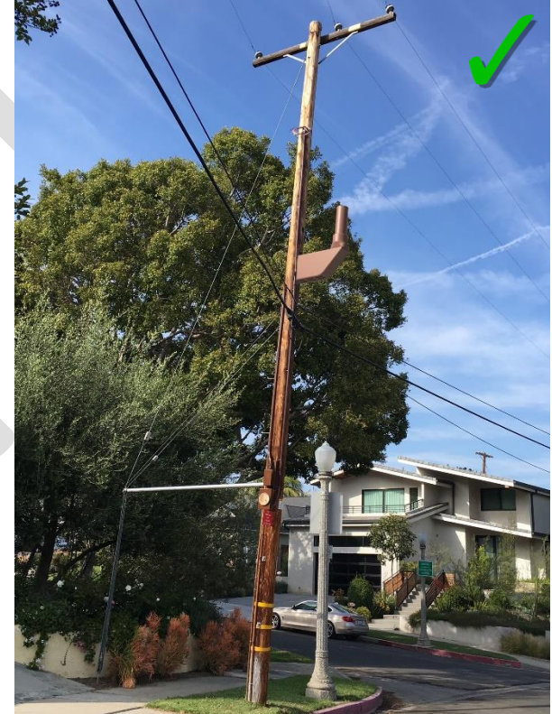
Figure 32: Successful example outside Calabasas; equipment is minimal, and painted to match pole.
