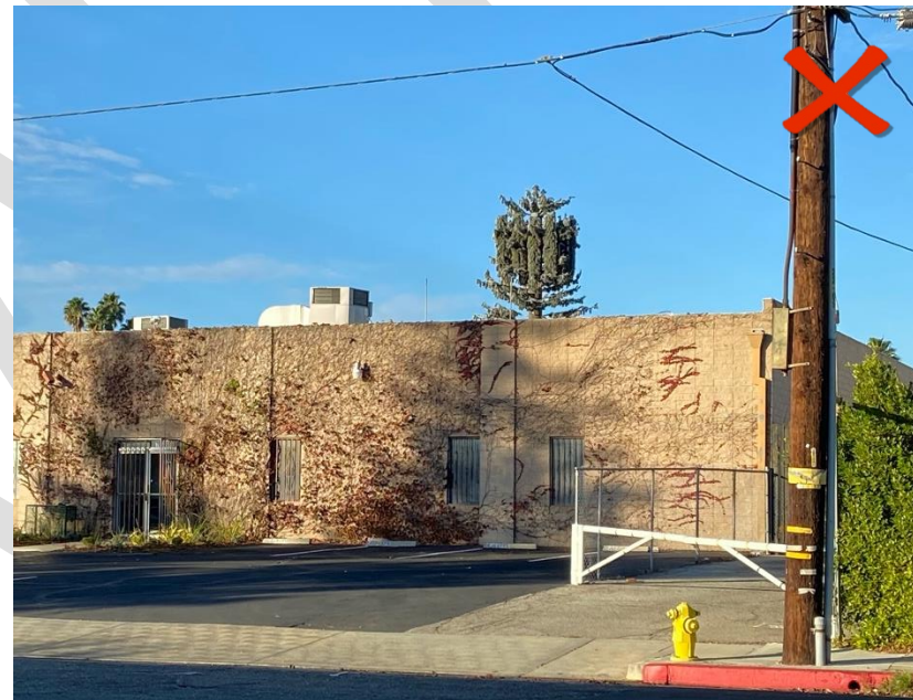
Figure 11: Unsuccessful example outside Calabasas; tree design adequately screens antennas, but the facility does not blend in with surrounding environment.
