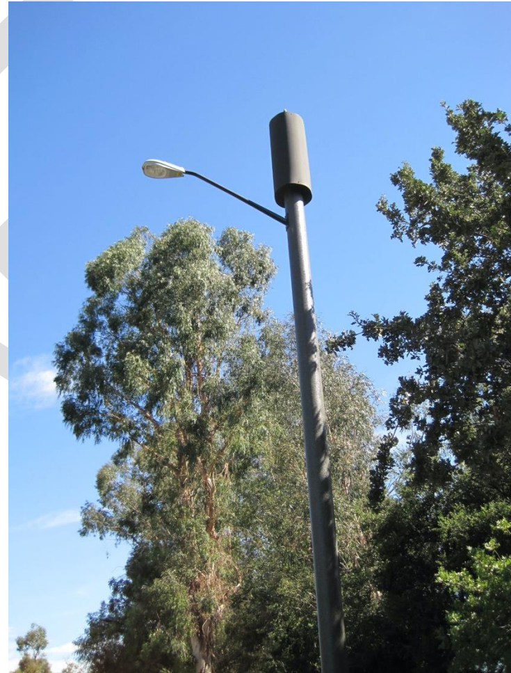
Figure 1: Example of stealth facility in Calabasas, mounted to light pole in Public Right-of-Way.
