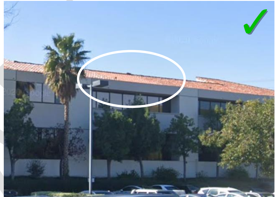
Figure 7: Successful example in Calabasas; faux roof tile element screening facility located on top of the building. Design closely matches surrounding tiles.
