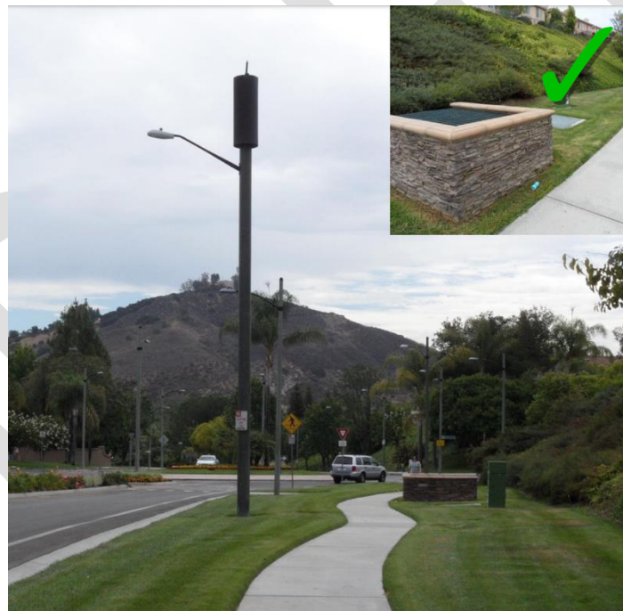
Figure 23: Successful example in Calabasas; equipment concealed within radome ground mounted equipment screened behind rock wall enclosure.
