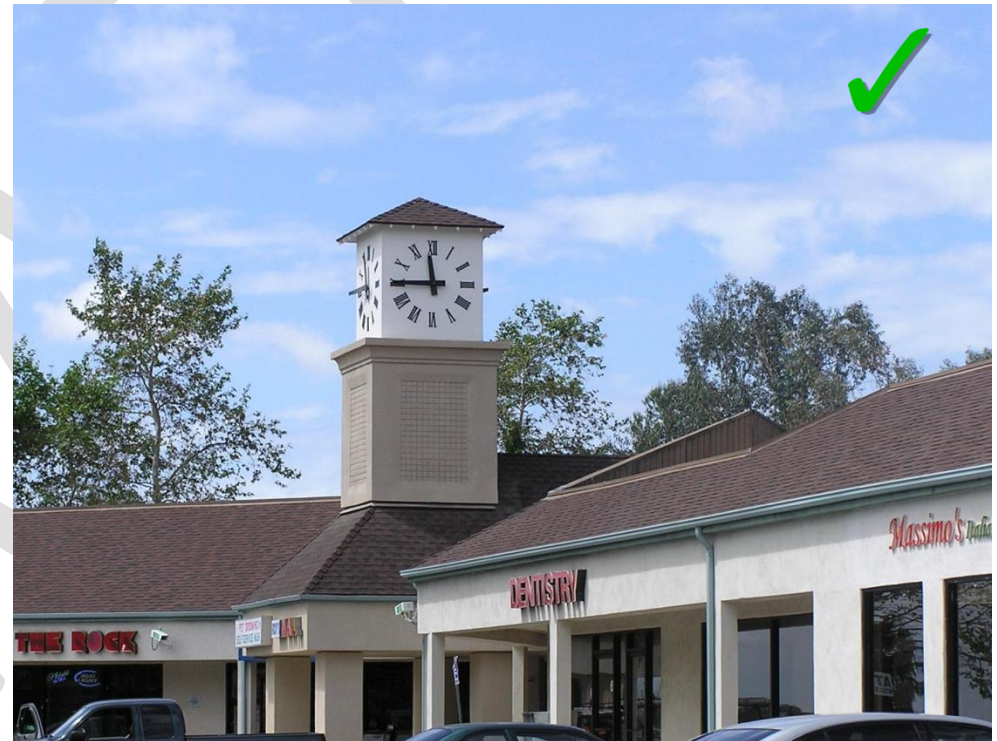
Figure 9: Successful example outside Calabasas; all equipment concealed within feature and is architecturally compatible with existing roof.
