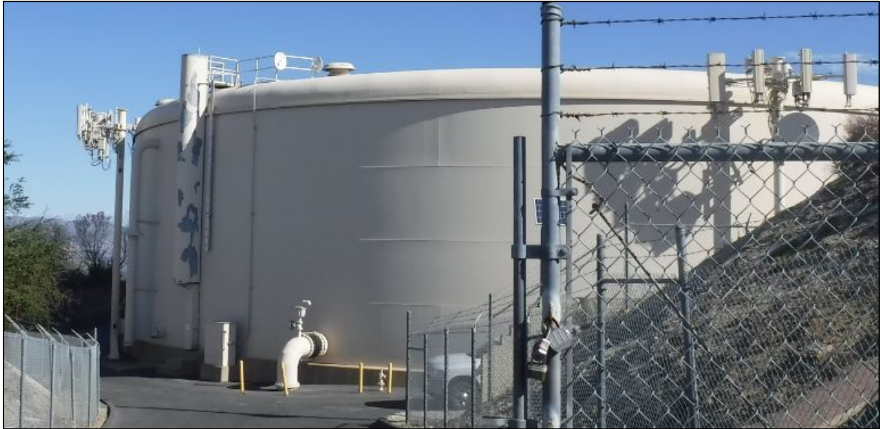
Figure 1: Photo of project (Source: Applicant submitted Photo).
