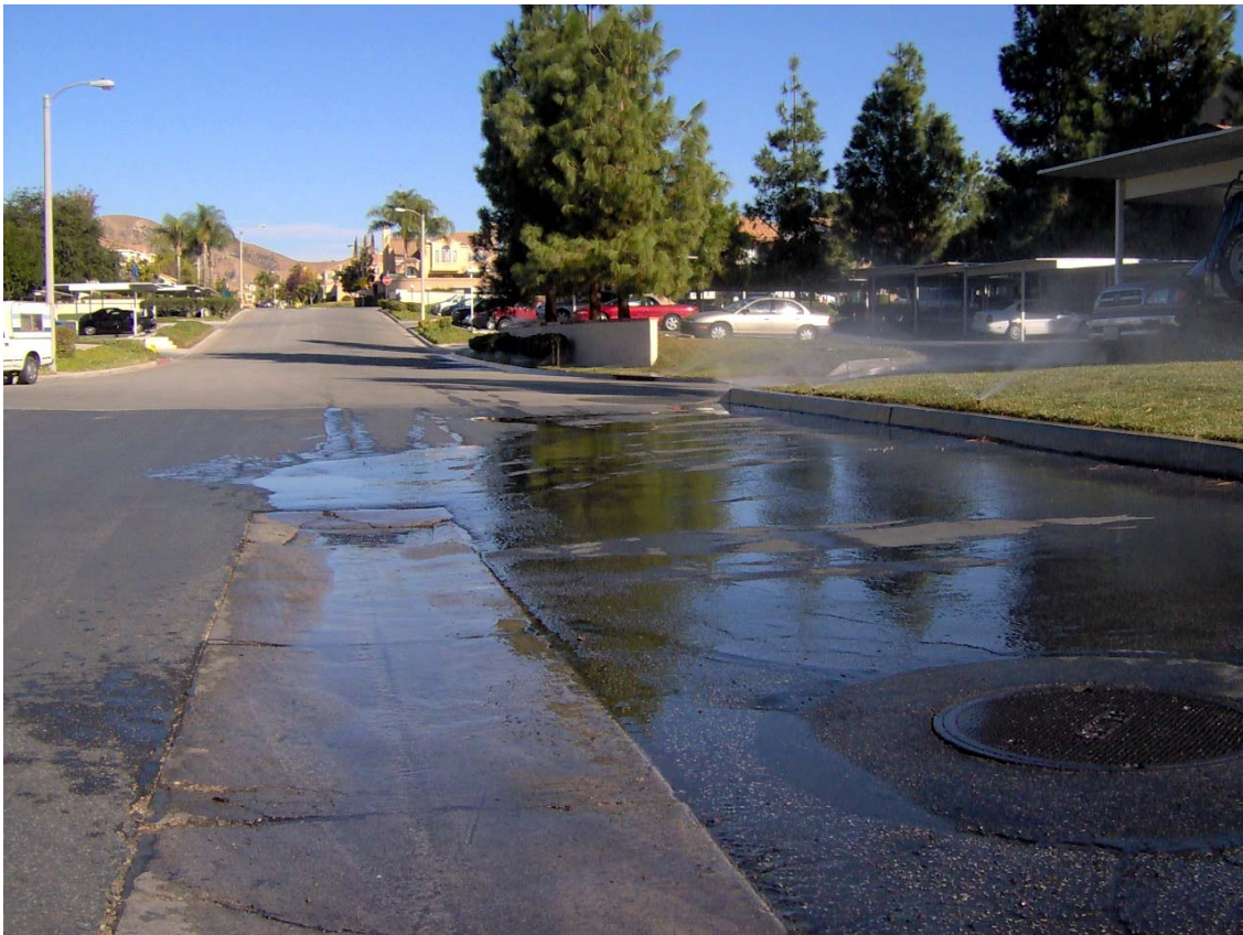
Image 3: Irrigation runoff at south end of Poppyseed lane entering a storm drain
