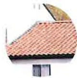
• "S" Tile Roof
