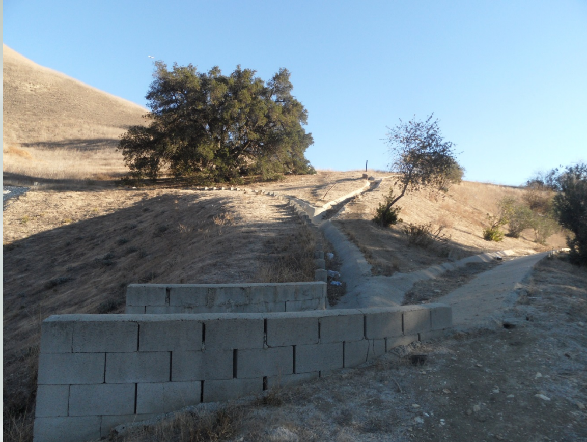
Facing east from subject site
