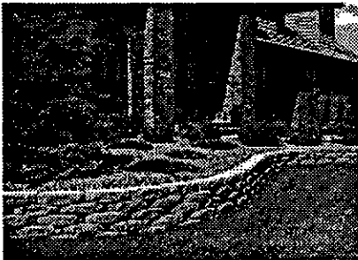
Stone retaining walls to be used for slope bank retention and decorative landscaped planters
