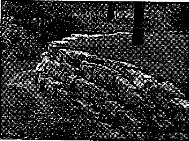
Natural stone retaining walls to be used for slope bank retention and decorative landscaped planters
