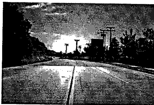
Steep slopes and unsightly utility lines east of Freedom Drive
