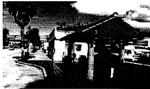
Bus stop shelter should be of simple design with mission tile roof, heavy timbers and stone or wood support posts
