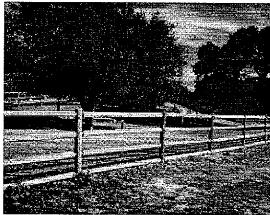
Turned post and rail fences used along road. Light gauge wire mesh should be installed between ground and lowest rail to prevent small animal from crossing
