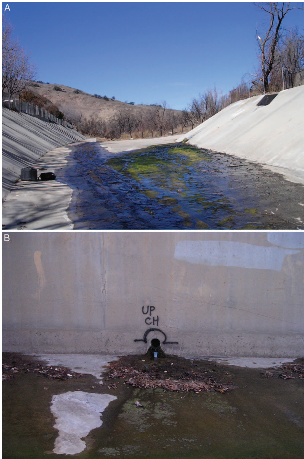
Figure 3. Photographs showing the transition zone between open space and the lined section of Las Virgenes Creek (A) and a weep hole in the lined section of Las Virgenes Creek (B).
