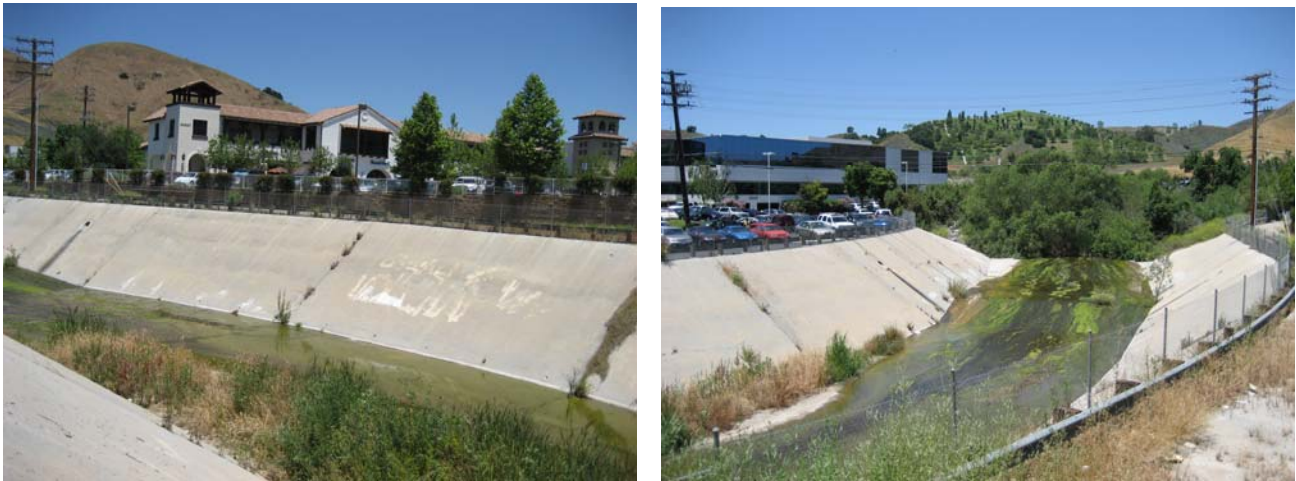
Concrete Channel built in 1977
